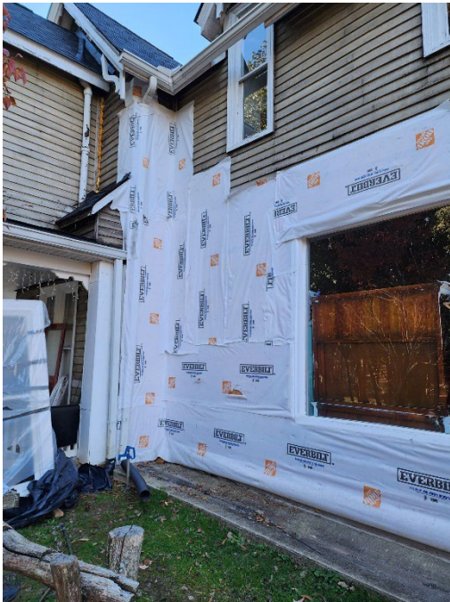
Inside corner with water filtration problem
